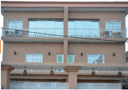
Bâtiment abritant GERIA Building housing GERIA
